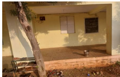
ZP School before the painting project
